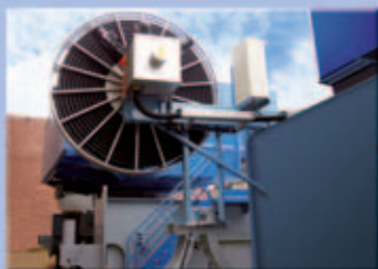
External power supply from on-shore mains source
