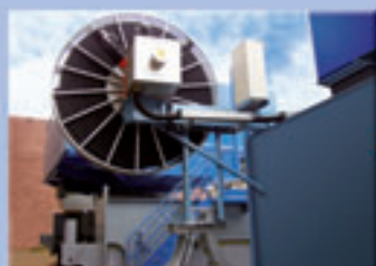
External power supply from on-shore mains source
