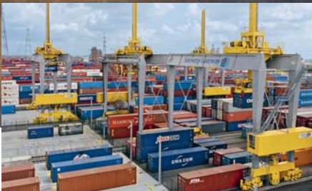
... where they are stacked by Gottwald ASC Automated Stacking Cranes and then loaded onto rail and road vehicles.
