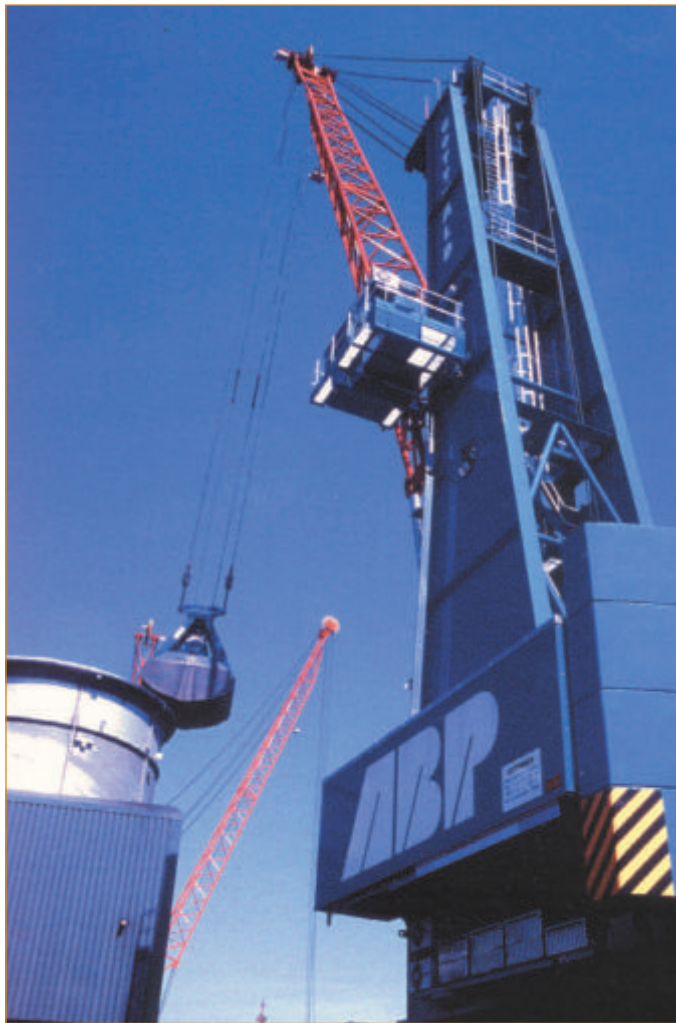
HMK 280 EG discharging coal for power generators at the Humber International Terminal, UK.
